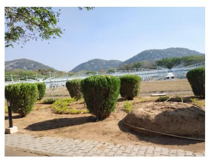
Yagi-Uda antennas arranged in a 32 x 32 matrix over an area of 130 m x 130 m. The two sets are colocated with pairs of crossed Yagis mounted on the same set of poles. The array is aligned along the geomagnetic axes to enable the radar beam to be transverse to the Earth's magnetic field for ionospheric backscatter application. The array of either of the polarizations is illuminated using 32 transmitters of varying power, each feeding a linear sub-array of 32 antennas.
